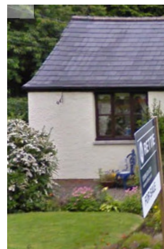
Detailing of applicant dwelling note traditional painted harl render, exaggerated kick to base of roof + original slate with bedded ridge tiles
